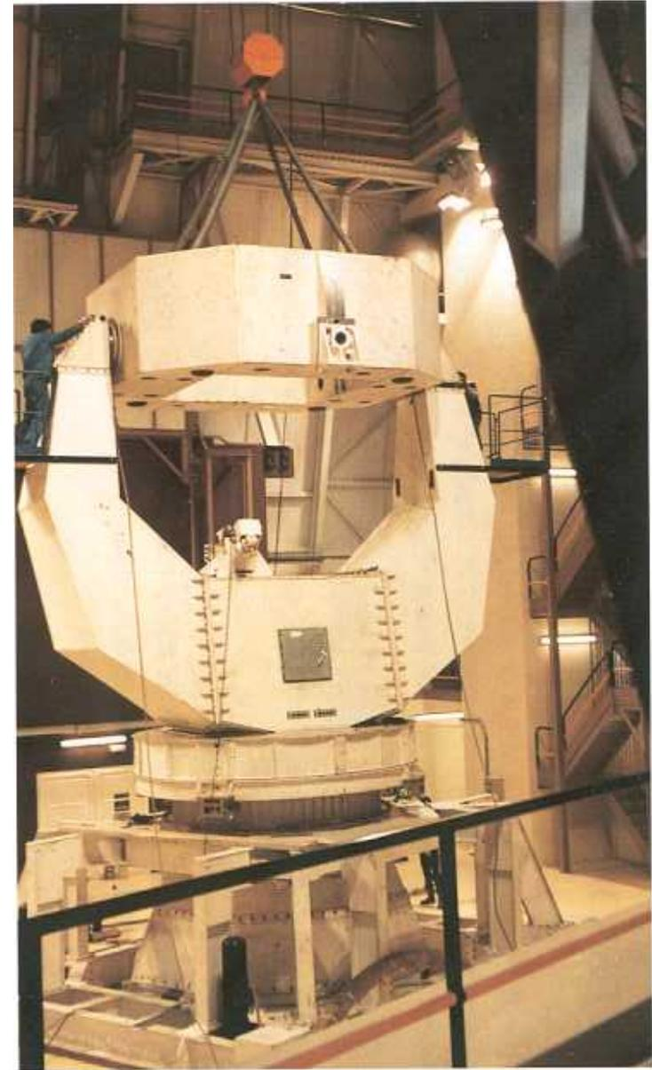
**Fig. 5.10:** Assembly of the Antenna 4 telescope mount. On the left-hand side one arm of the fork is being mounted, on the right-hand side the elevation frame, which has a weight of 16 tons, is being integrated. The latter interfaces with the central hub of the reflector.
