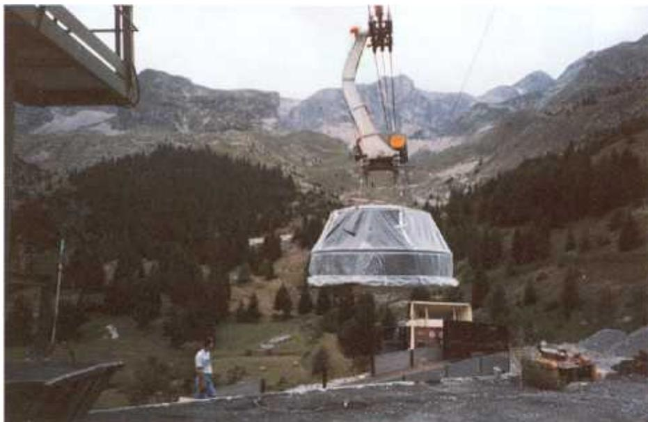
**Fig. 5.8 :** The transport of the central hub from the lower cable car station to the Plateau
