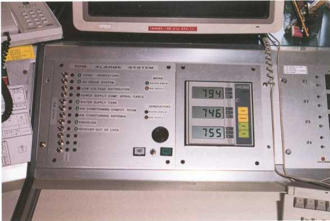
**Fig. 3.3:** Alarm control panel at the operators' desk.
