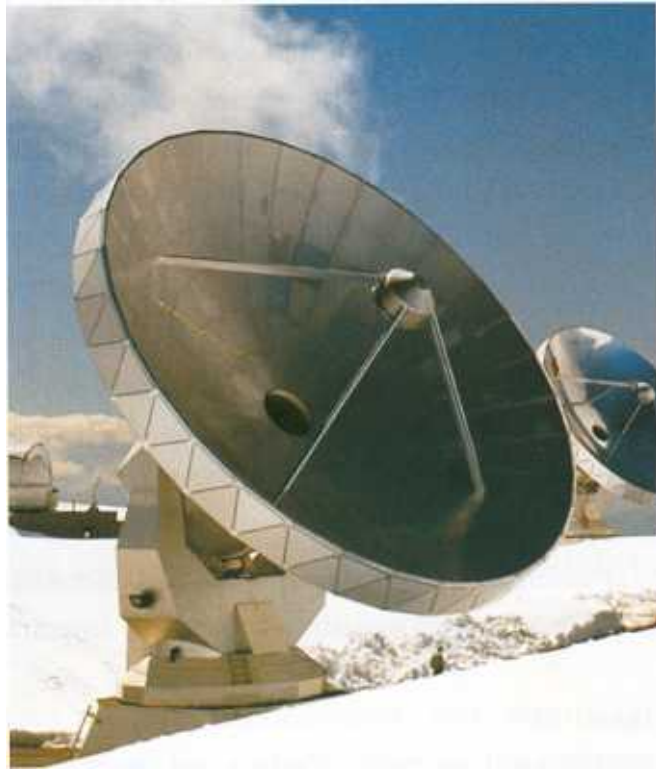
Fig. 4.1 : Antenna 5 with its reflector made of 176 aluminium panels.
