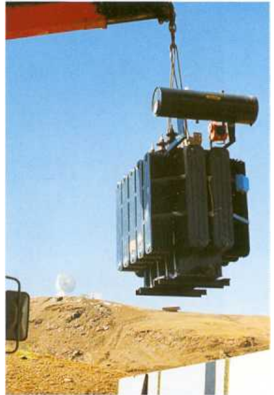
Fig. 3.4 : Removal of the old pyralene transformer
