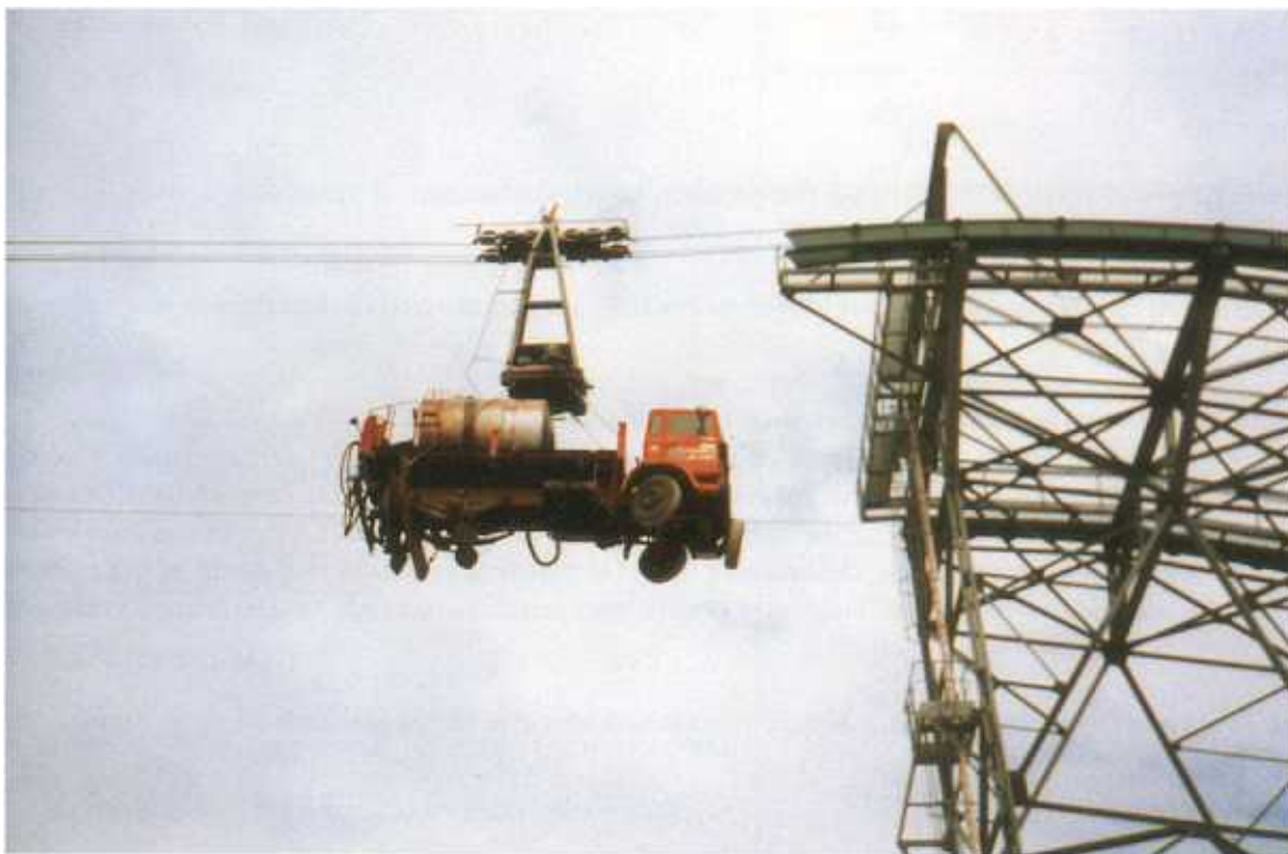
What had to be organised to asphalt the tracks.
