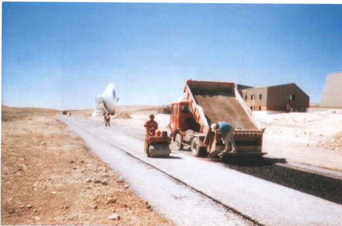
Asphalting the tracks.
