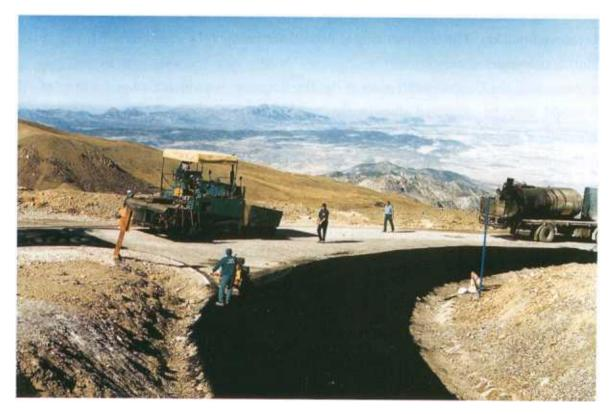
Fig. 3.2: Repair and pavement of the access road to the telescope
