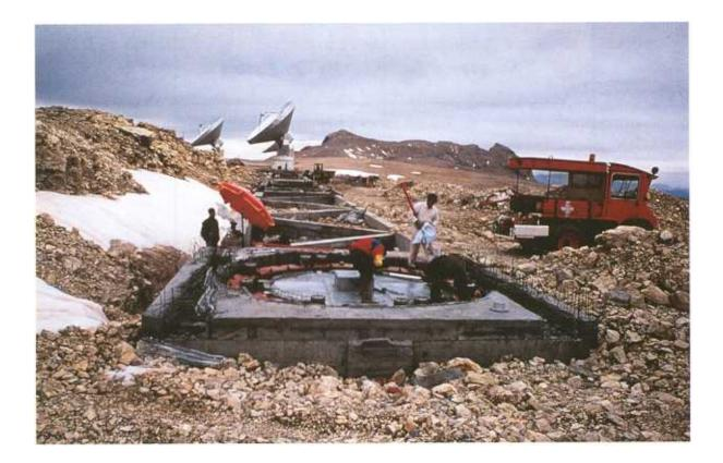
Fig.4.1: Work on the E-W track extension from 288m to 408m, including the new stations W20, W23, and W29
