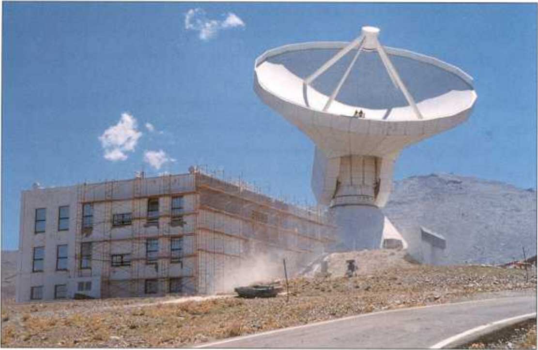
Fig. 3.7: The control building during the maintenance and repair work at the outside walls
