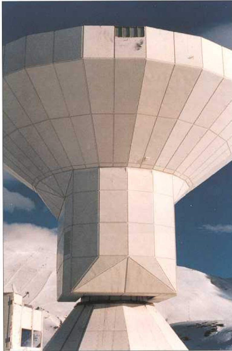
Fig. 3.6: Damage of the cladding of the 30m-telescope caused by a lightning. One of the outside panels was affected by the impact of the lightning.
