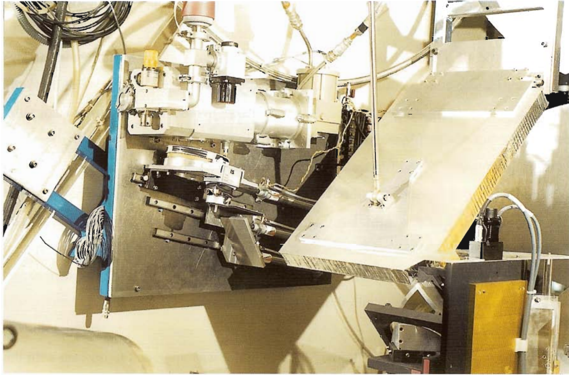
Fig. 3.8: The new calibration system in the refurbished receiver cabin.
