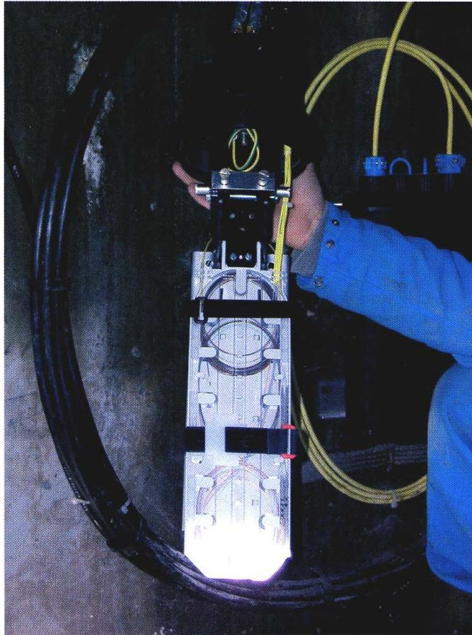
**Fig. 4.8:** View of the waterproof fiber optic connector installed in the stations. At this, 6 fibers are actually arriving at each station. This number can be increased to 10 if future generations of receivers require this.
