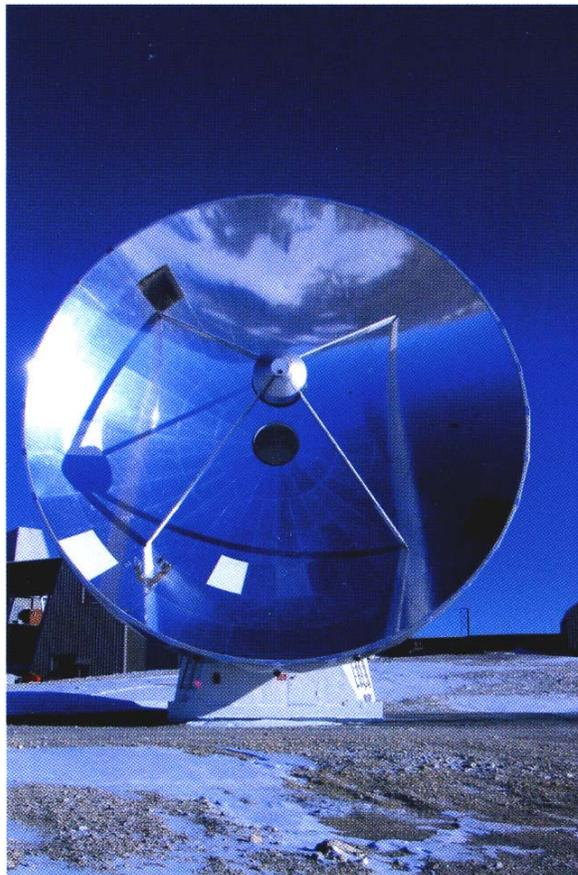
**Fig. 4.7:** The surface of Antenna 1 with three panels replaced during the summer maintenance. These are carbon fiber panels with a reflective layer of silver paint, and a protective cover of white paint.
