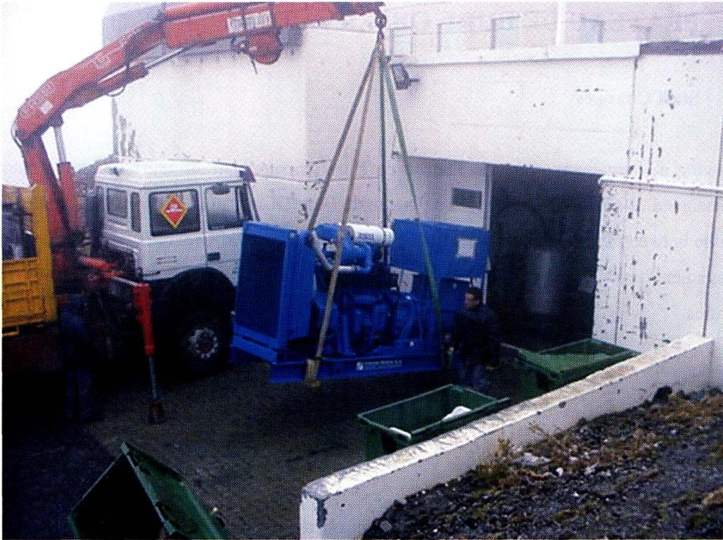
**Fig. 3.9:** Installation of a new Diesel generator
