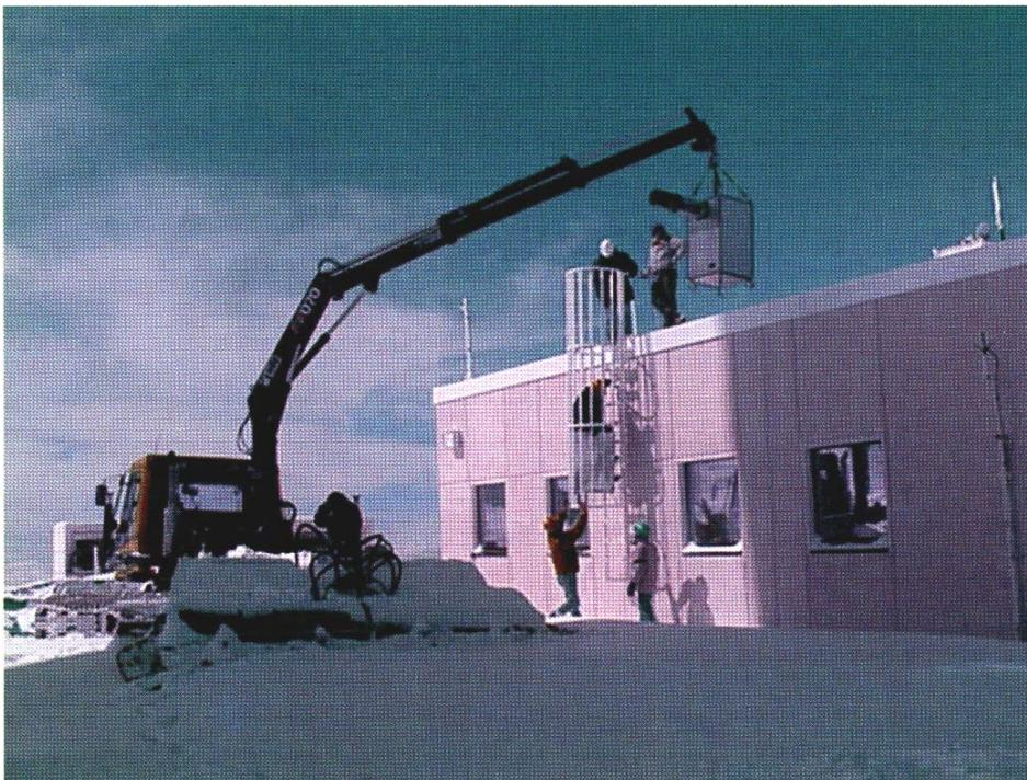
**Fig. 3.5:** Installation of the taumeter on the roof of the control building.
