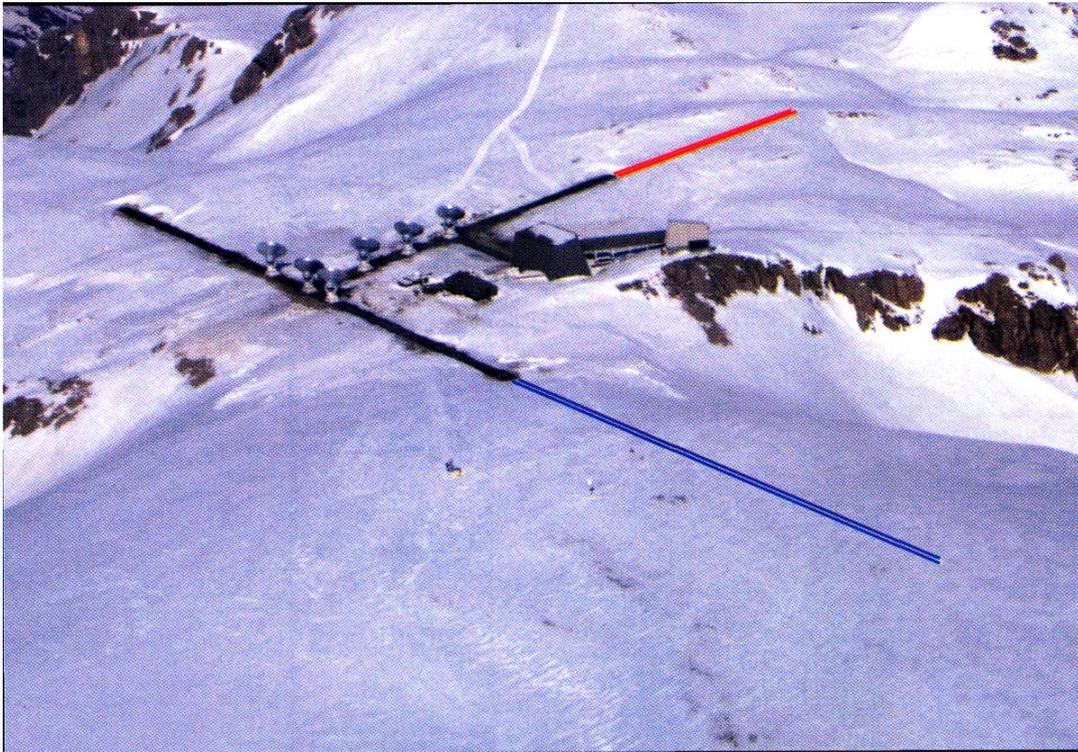
**Fig. 4.5:** Aerial view of the Plateau de Bure Interferometer in its D configuration. The northern track extension (red), which is awaiting completion, and the planned extension (blue) of the eastern track are expected to double the current angular resolution capability of the interferometer: astronomical targets will then be mapped with a 0.3 arcsec resolution at the frequency of the CO(2-1) line.
