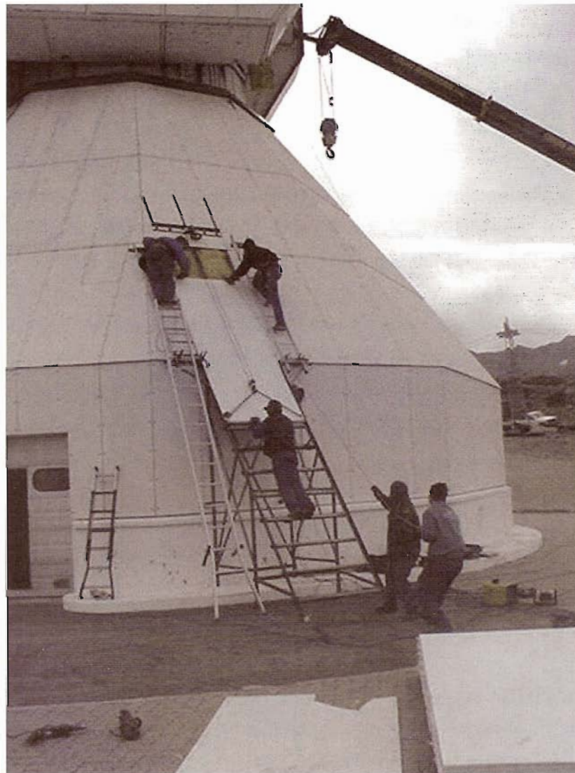
Fig. 3.7: Replacement of broken eternit plates at the 30-m telescope
