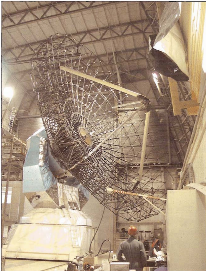
Fig. 4.1: The back structure of Antenna 6, as of August 31 st , 2001. Surface panels were placed in September and October, and also the thermal insulation of the yoke.
