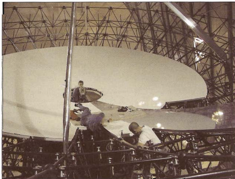
Fig. 4.3: The surface of Antenna 6 after three weeks of panel assembly work. Surface fine adjustments will have to await holography measurements on astronomical masers.
