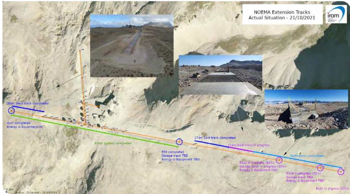
Situation of the track construction site on 21/10/2021.
