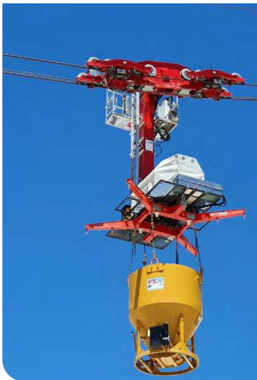
Left: Aggregate bucket adapted to the material ropeway.
