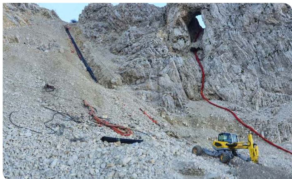
Realization of the works on the 20kV line.
