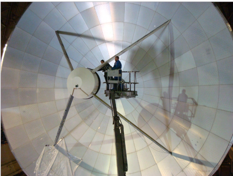
Inspection of the subreflector of a Plateau de Bure antenna during regular maintenance operations.
