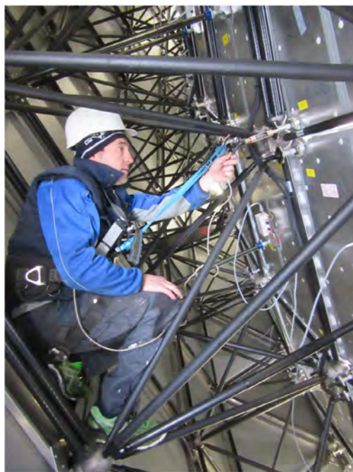
A technician aligning surface panels in the dish of a NOEMA antenna.
