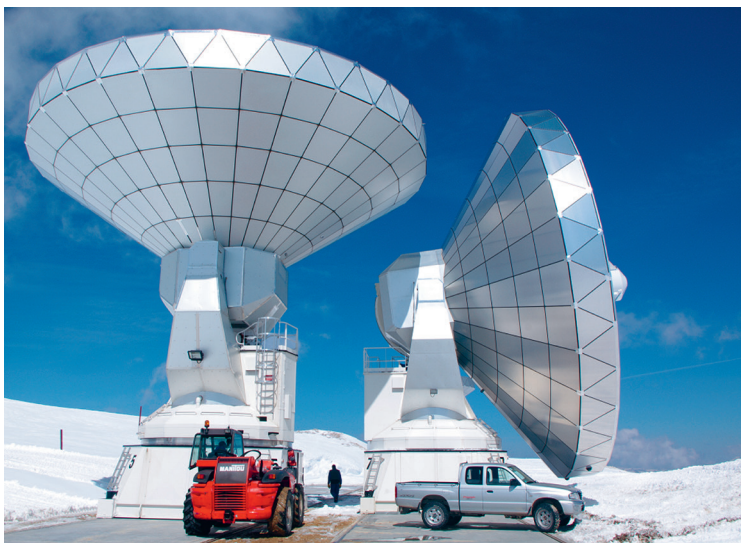
IRAM staff taking advantage of the northern bypass track to relocate two antennas for an array configuration change.
