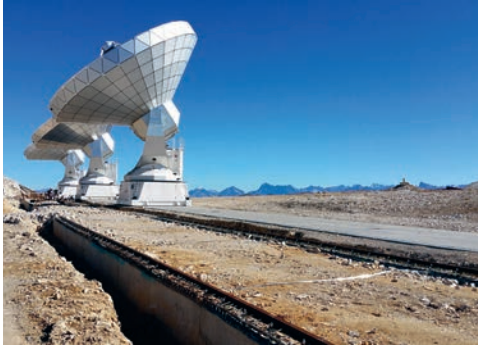
Top: NOEMA antennas performing science observations during the construction of the northern bypass track.
