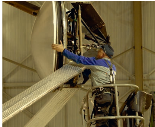
Technician verifying the subreflector mechanics in the frame of the regular antenna maintenance activities.
