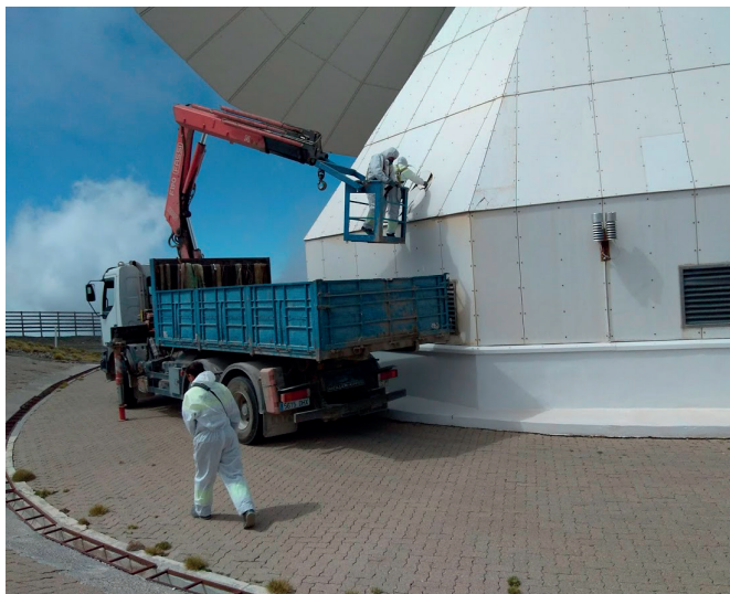
Replacement of fibre cement panels (Eternit) in the 30-meter antenna tower.
