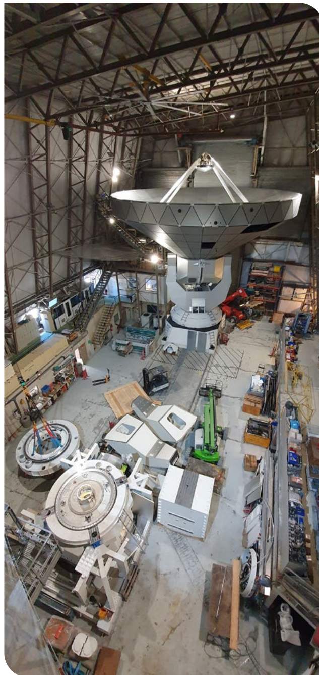
Construction of Antennas 11 and 12.
