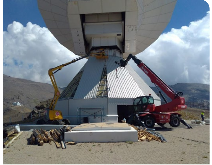
Installation of the new asbestos-free cladding.
