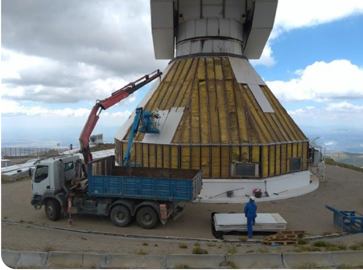
Removal of original fibre-cement plate.
