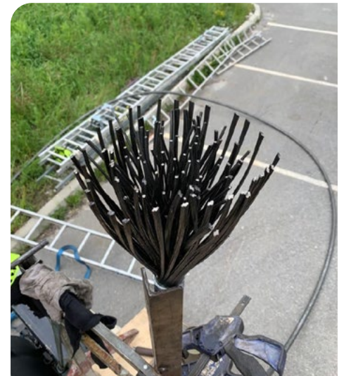
Section of the old cable composed of numerous strands.
