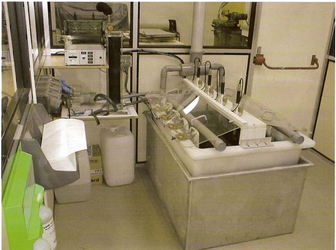
Fig. 5.16 : The new installations for electro-forming
