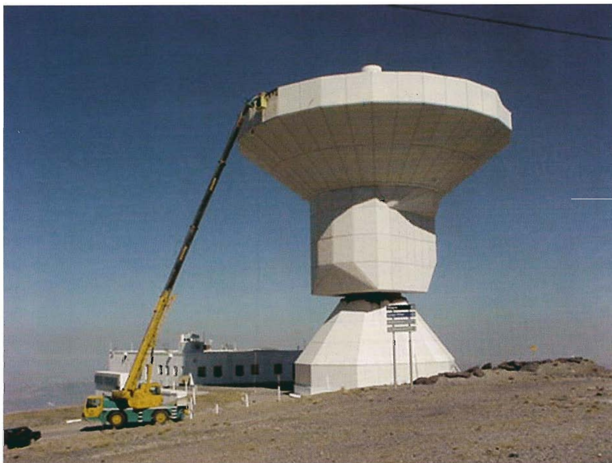
Fig. 3.6: Repairing the backstructure of the 30m telescope
