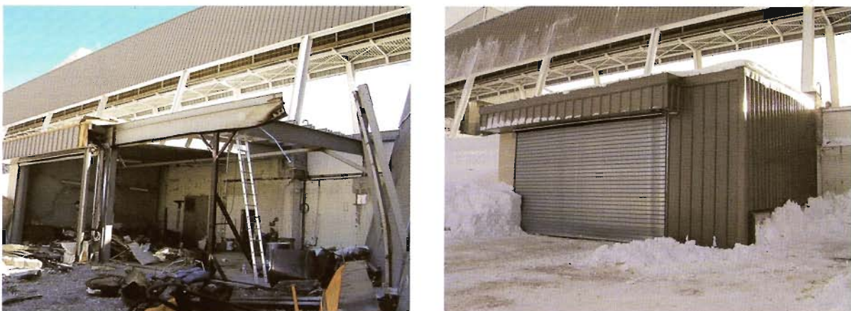
Fig. 4.6: The Ratrack garage before and after refurbishment
