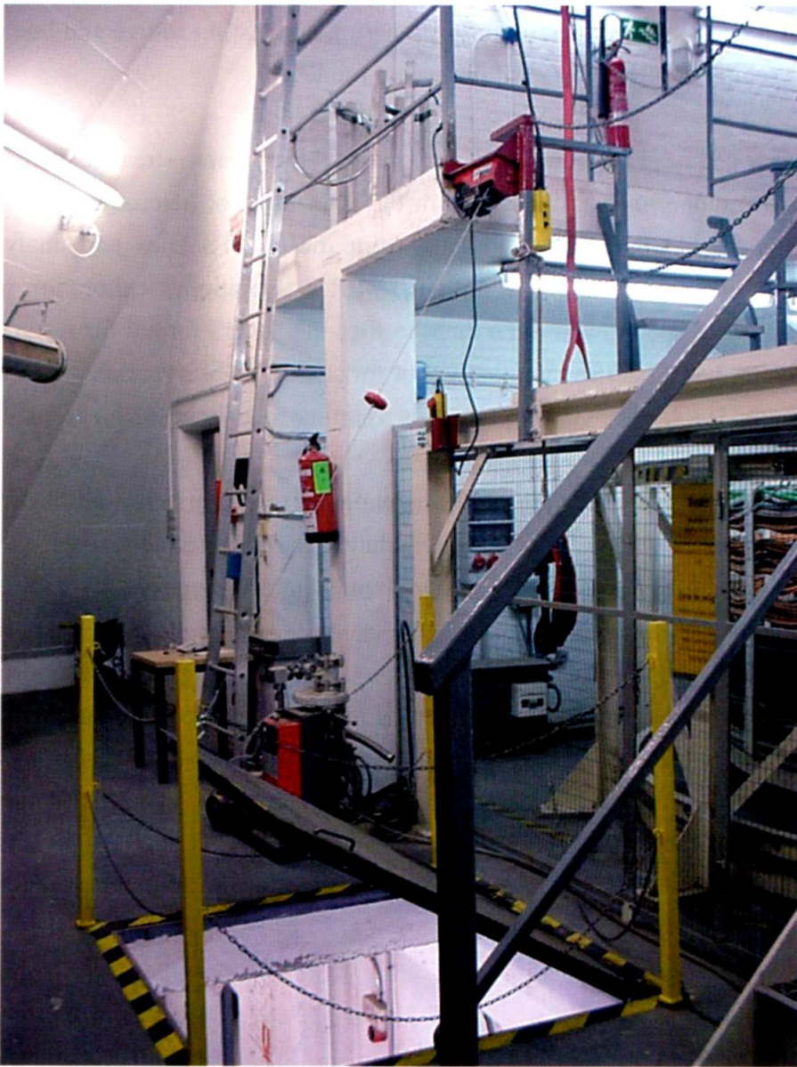
Fig. 3.6: The trap-doors in the telescope tower are now operated by motors.
