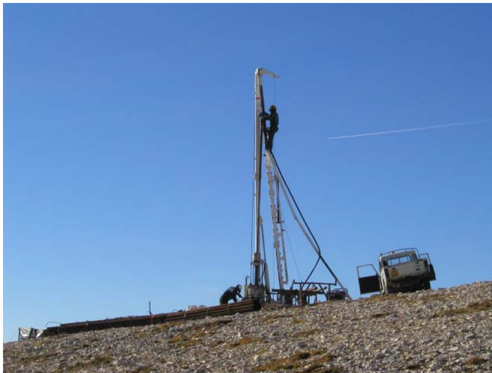
Fig. 4.5: View of the drilling machine on the Plateau de Bure
