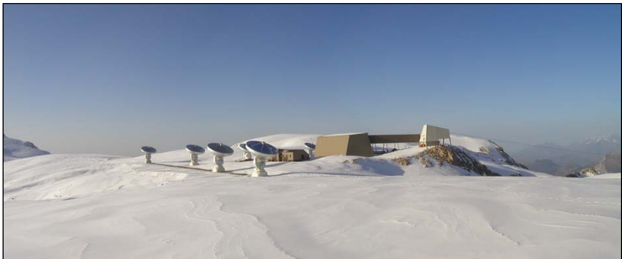
Fig. 4.1: The Plateau de Bure Observatory: the 6-element interferometer in an intermediate configuration with the main building and the hangar for antenna maintenance.
