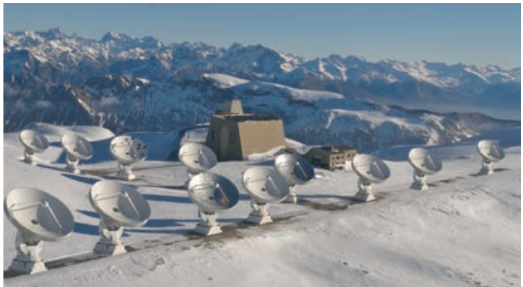
Photomontage of the Plateau de Bure interferometer with the six additional antennas planned in the NOEMA project.
